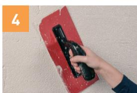
Finishing must continue before the skin dries. Finish (float) the levelled area in circular strikes to further fill and even out material. Use harder pressure to fill low spots. Work in larger, lighter strokes as material levels out. Use a clean bucket of water and a sponge to clean and keep the plastic float moist.
