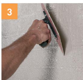
Levelling must continue before the skin dries. Working from the ground upwards, hold the plastic float against the surface so that the leading edge is raised and angled at approximately 45 degrees. This process can be done in pairs, with one person levelling as the other continues delivering product to the wall. Push the material across the surface to fill joints and low spots. This process should broadly distribute and level the roller applied texture before it sets.
