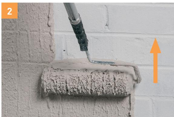
Stir contents of *Dulux Texture Full Cover Roll On* with a broad flat paddle using an up and down scooping motion. Pour contents into a deep roller bucket or tray. Using a *Full Cover Texture Roller*, load the roller, then deliver material to the wall in vertical strips to 1/2 to 3/4 metre from the ground upwards with a smooth steady action. Avoid rolling downwards as excess material may fall from the roller. After 4-5 roller widths have been applied the levelling process should be commenced.
