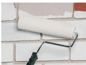
Applying 1 coat of *Dulux Texture Primer™* is recommended to condition the surface and aid application of successive coats. Areas that aren't accessible by roller, should be cut in with a brush. Apply 1 coat of *Dulux Texture Primer* with a roller and allow 4 hours dry time before applying *Dulux Texture Full Cover Roll On*.
